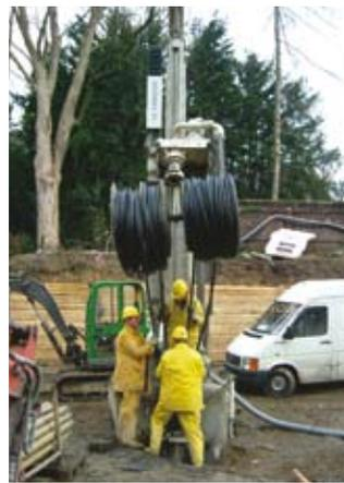
Fig.7: Sonda RAUGEO PE 100
